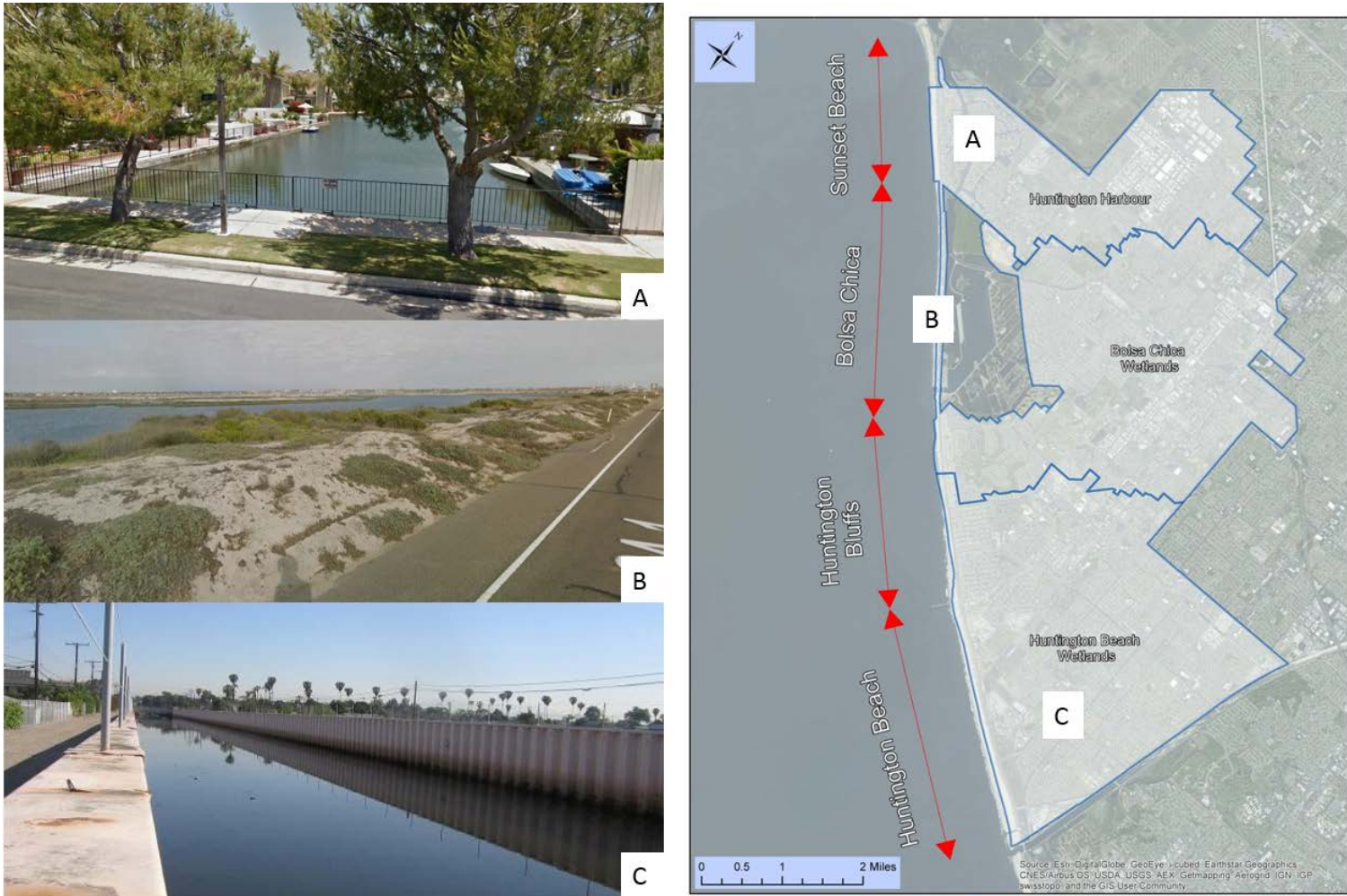
FIGURE 1 EXAMPLES OF INLAND WATERWAY COASTAL STRUCTURE EVALUATED FOR TIDAL FLOODING
